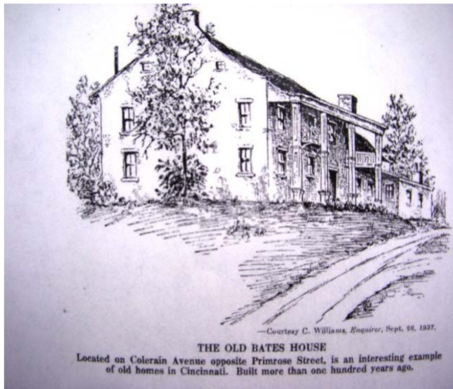
Mount Comfort, the old Bates place, stood near the former Cincinnati Workhouse. Torn down, 1930s.
