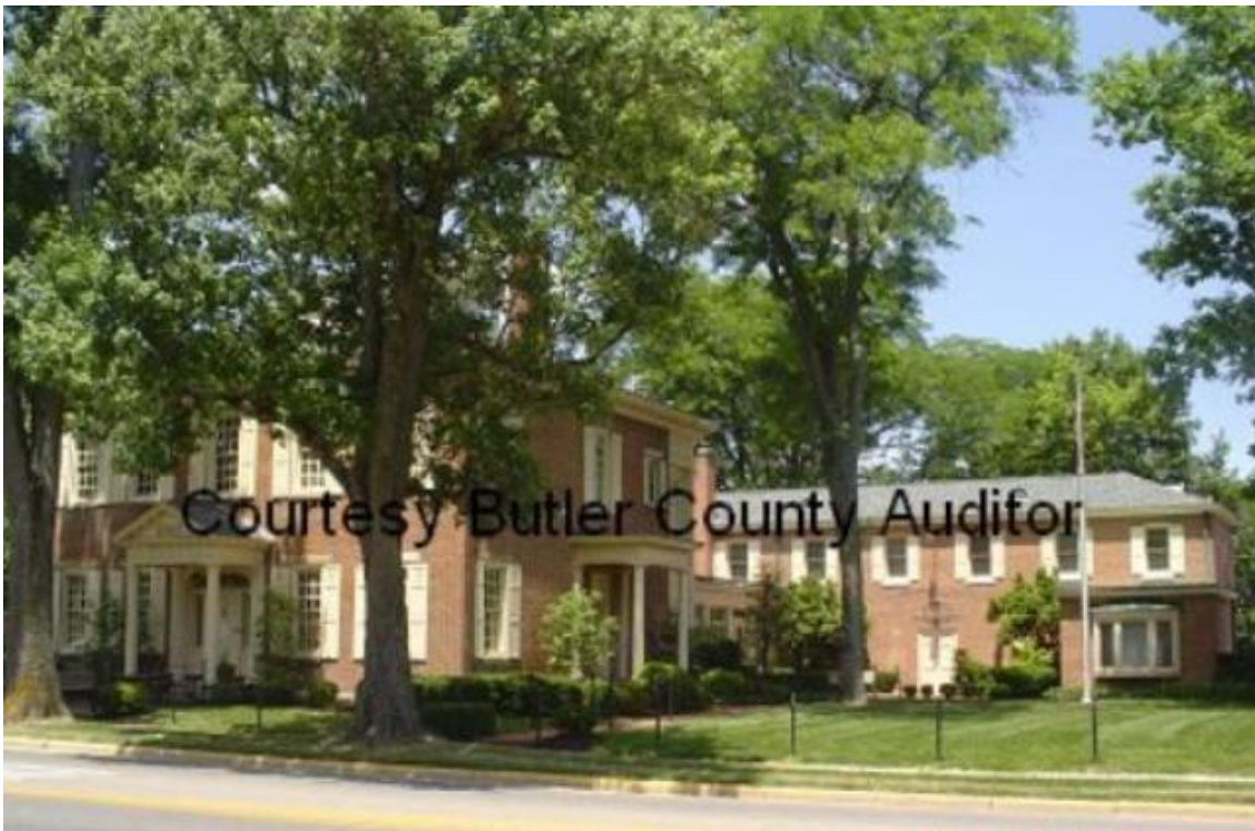
Beta Theta Pi House, East High Street, Oxford, Ohio. Section on the left was the home of the Olivers; extensively remodeled.
