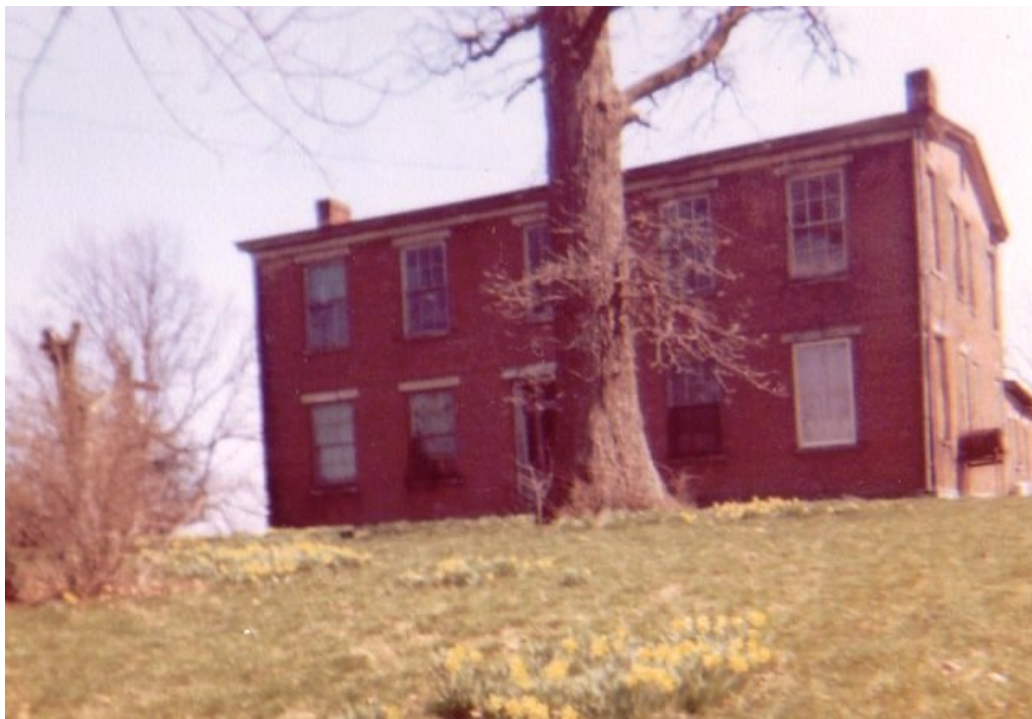
Forest Home, 1984, just prior to demolition.
