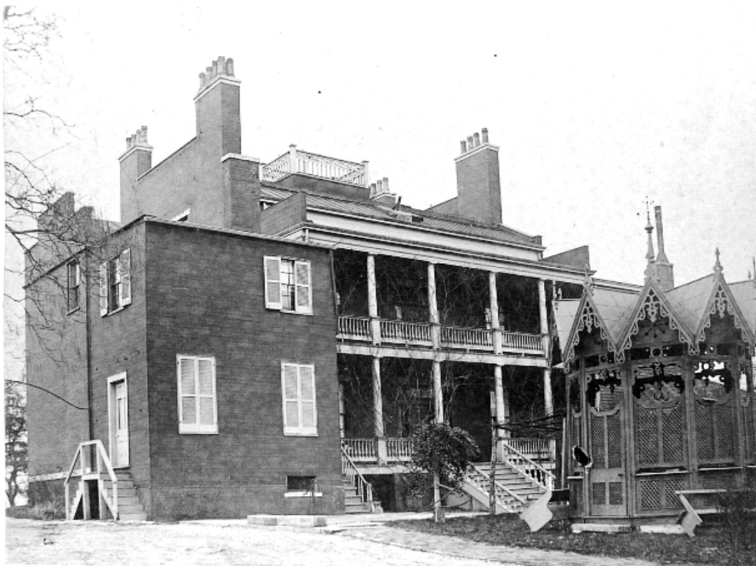
Beech Grove, rear view showing kitchen wing, portico, gazebo and 21 chimney caps.
